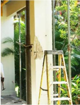
A significant restoration project is slated to begin this December at Bonnet House as concrete arches, columns and beams in the courtyard undergo rehabilitation. Cracks and flaking became much more noticeable over the summer and engineering analysis revealed that the deterioration was more than aesthetic and
